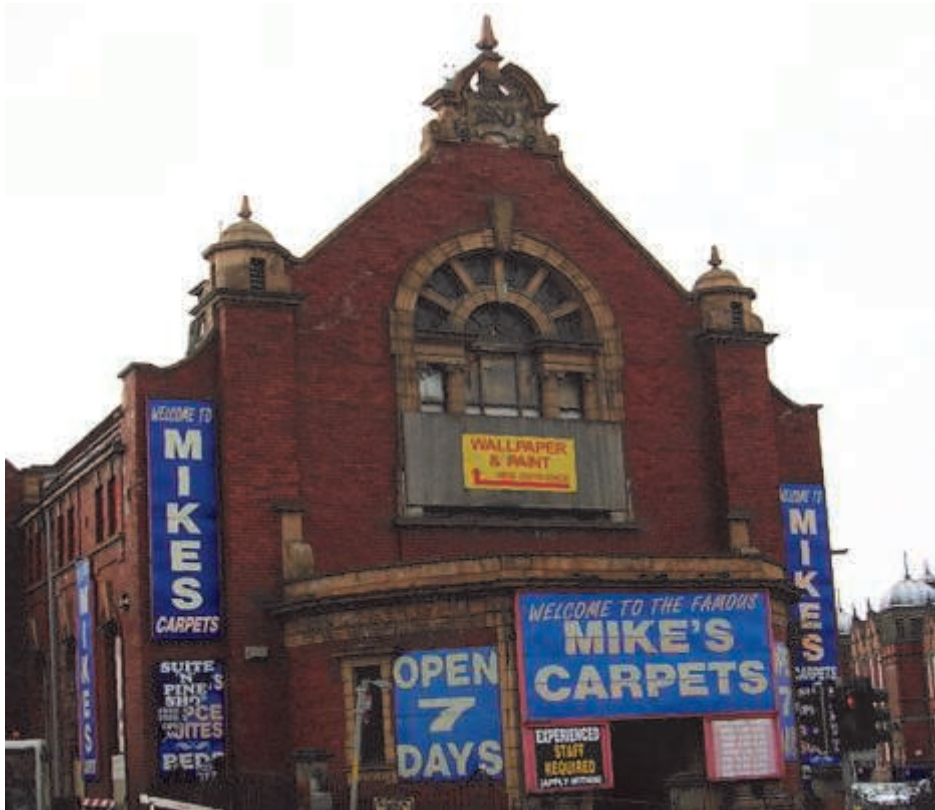
Former Methodist Chapel in Birmingham, now a Carpet Warehouse.
